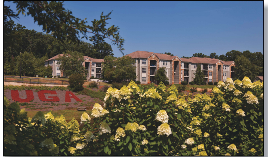
Acquired by Pierce Education Properties (PEP) in June, this 612-bed community in Athens, Georgia, represents an acquisition that meets the company’s investment criteria. The asset is 100 percent occupied for fall and is located in a highly stabilized university market.
